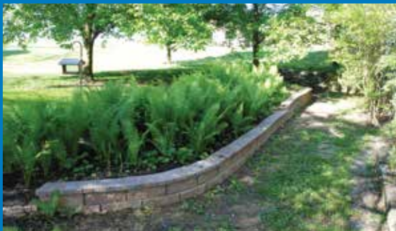
New retaining wall at the Myrick Center office.
