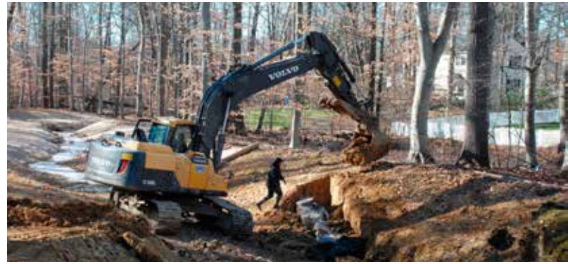
Installing a cross vane on Ludwig's Run.
