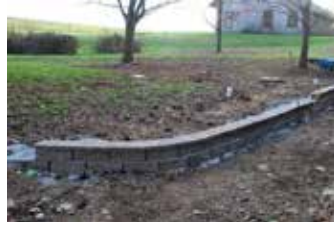
Scouts completing a stone retaining wall at the Myrick Center office.
